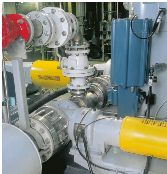
Fig. 28. ClO 2 mixing with chemical mixer.
